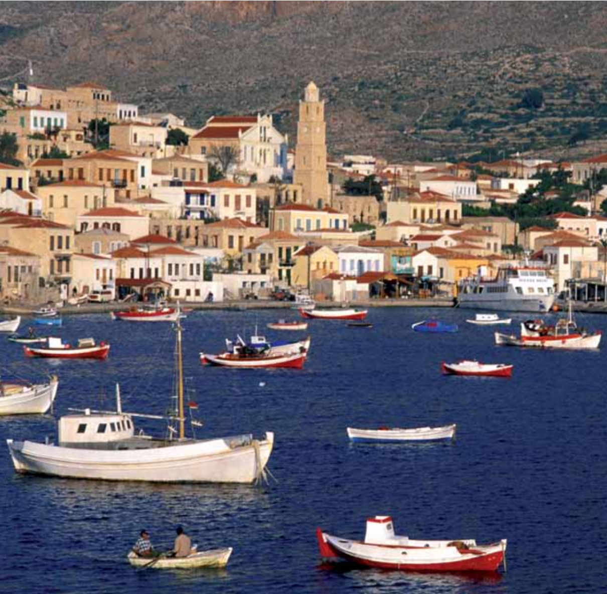
72. A view of Nimporio; the stone clock tower.
